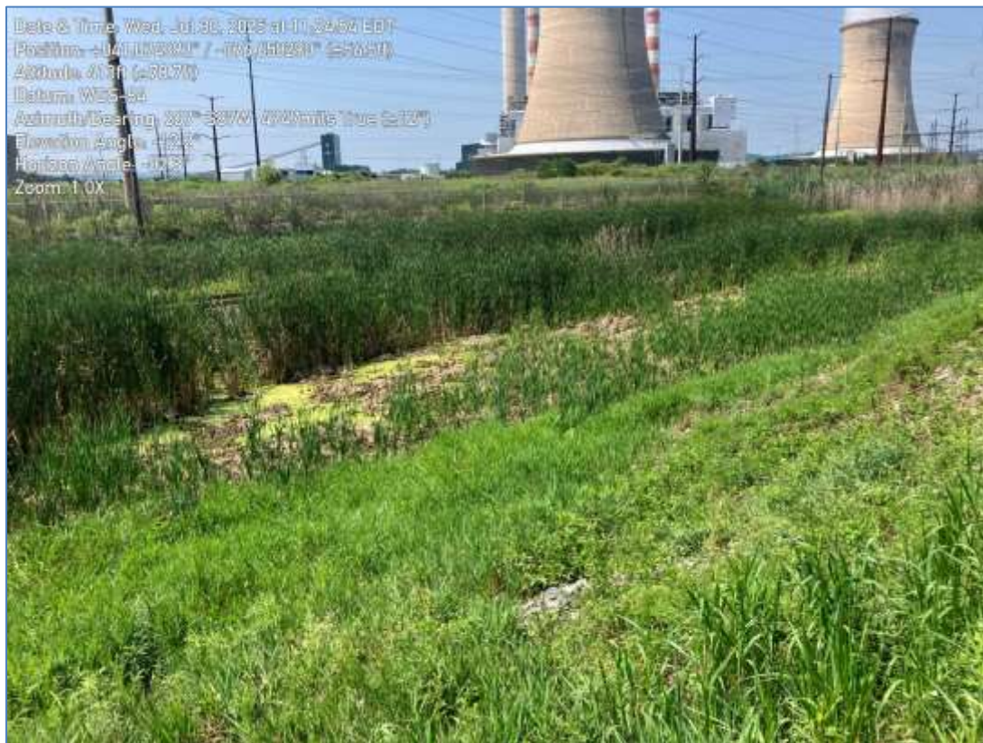
Photograph 5 – Evidence of ponding water at toe of western dike slope
