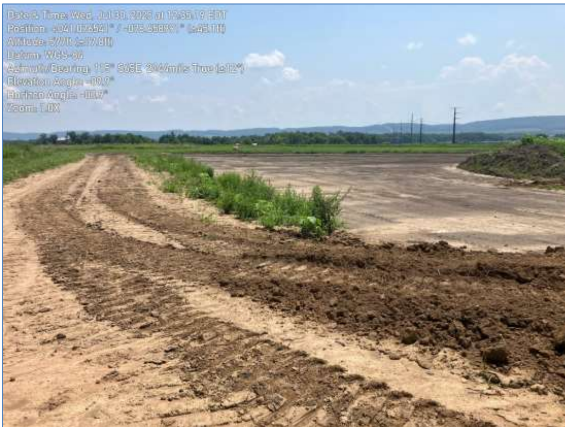
Photograph 26 – Fill placement and grading in Subbasin A
