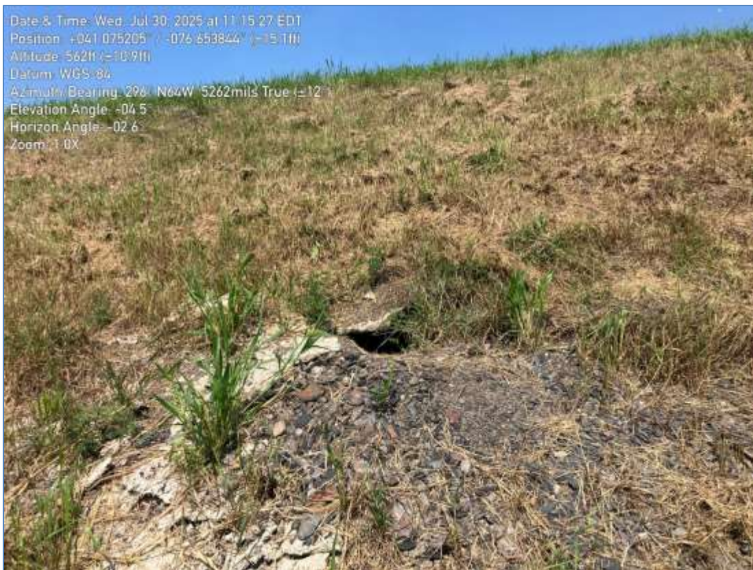
Photograph 4 – View of animal burrow hole on western dike slope
