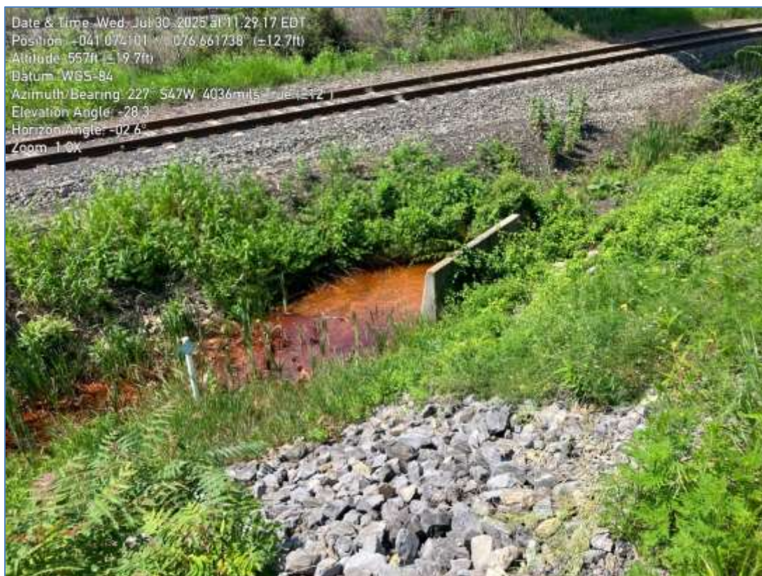
Photograph 6 – Iron oxidizing bacteria was observed in the sanding water at the toe of the western dike slope
