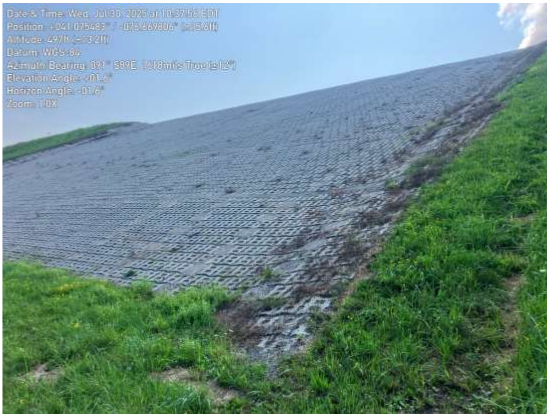
Photograph 25 – Overtopping protection installed at Subbasin C
