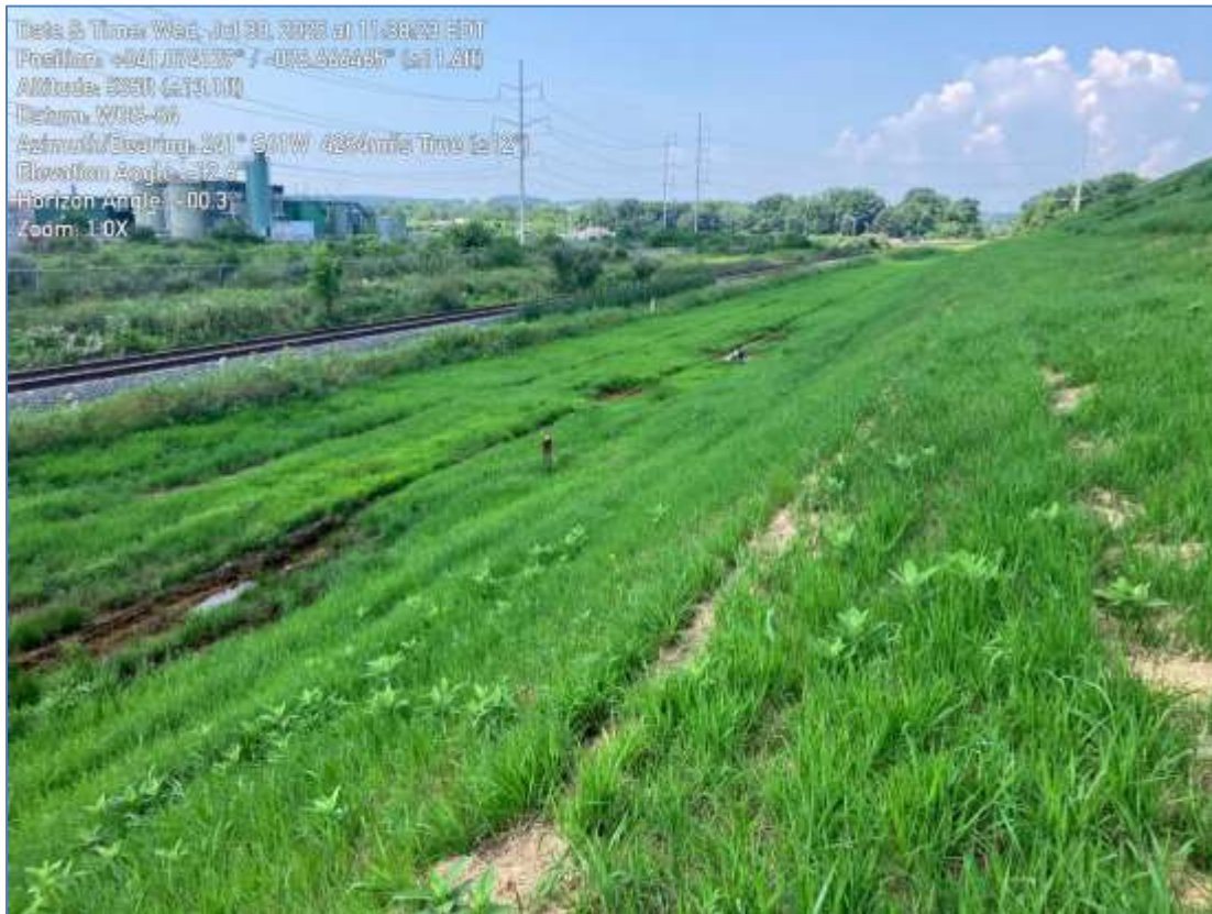
Photograph 7 – Ponding water at western dike slope toe, north of the pipe bridge
