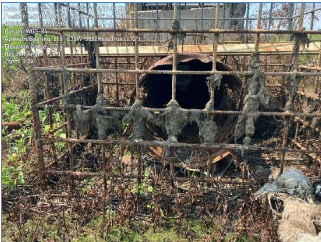
Photograph 20 – Subbasin B intake pipe with trash rack
