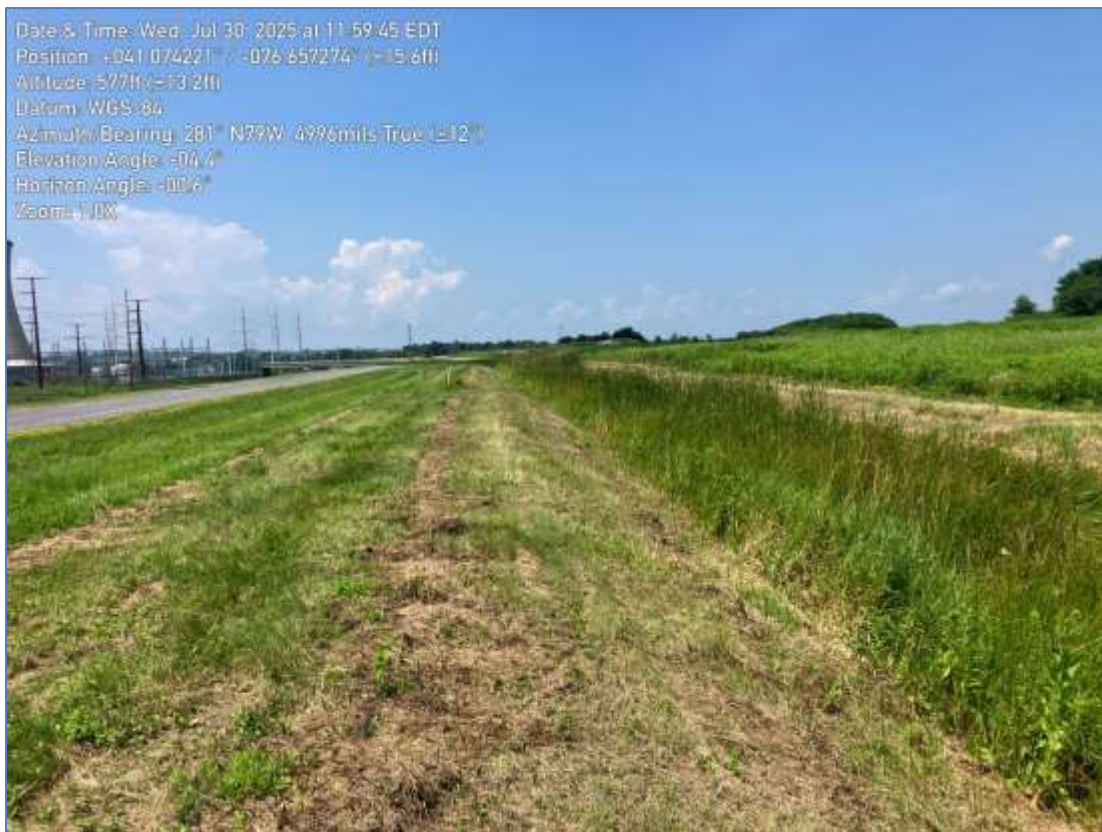
Photograph 8 – Western dike embankment crest and perimeter channel
