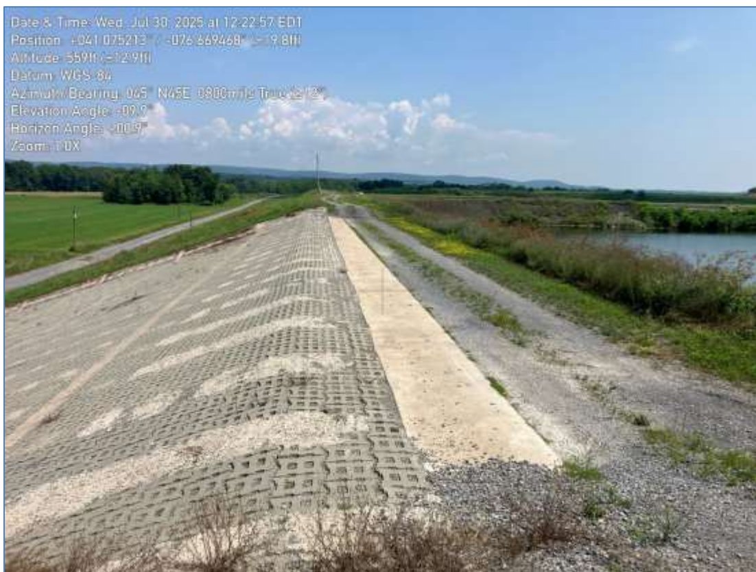
Photograph 24 – Overtopping protection installed at Subbasin C
